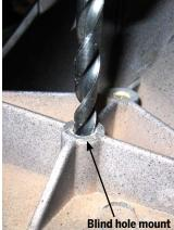
Figure 9: Drill Out the Mounting Hole
