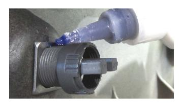
Figure 71: Apply Loctite 425
