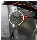
Figure 152: Motor Power Harnesses to PI Board
