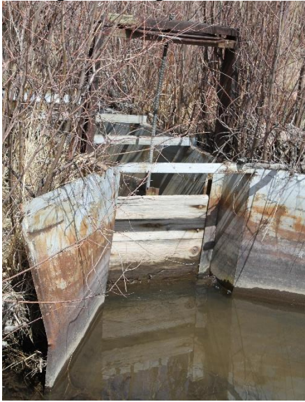
Headgate looking downstream
