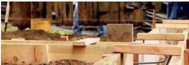
Top: Barn in lifted condition, placement of new concrete foundation; Bottom: foundation formwork
