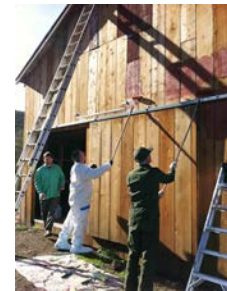
Painting repaired barn with NPS staff
