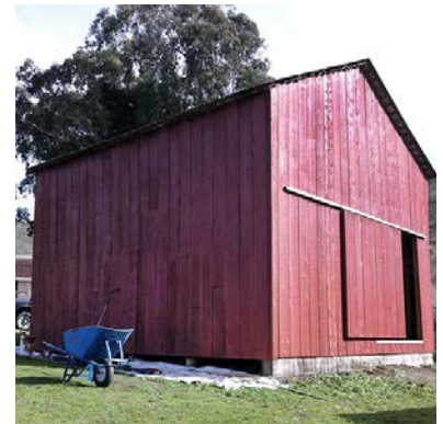
After: Repairs complete, building rear
