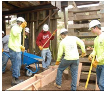
Foundation concrete placement
