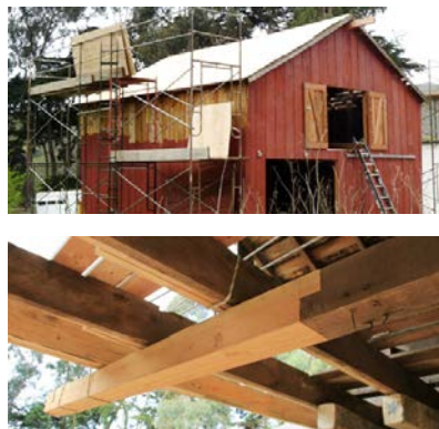
In Progress Top: New roof installation; Bottom: Splicing new wood members to historic
