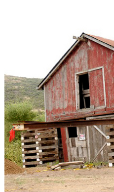
In Progress: Lifting entire structure to straighten, construct new foundation
