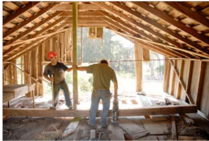
Straightening the structural frame after barn lifted off foundation
