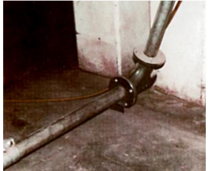
FIGURE #2 The HammerTek Smart Elbow™ sends "fines" from a line on the floor upwards to the cyclone. These fines are small food particles which are later recycled back into the production line. The upper end of this vertical run is shown in figure 3.
