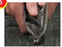
Cut an opening in the bag that suits the repair you are doing. For small spot repairs only cut a small hole in a corner. For larger repairs cut a bigger hole. Apply the resin to the damaged area by squeezing it out of the bag.
