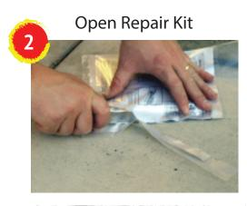
Feel the aluminum foil for the clip separator inside. Cut the foil along the edge to the outside of the separator clip.
