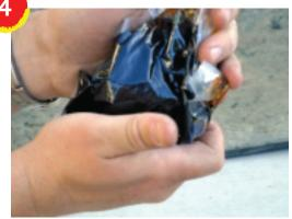
Mix the hardener and resin together for approximately 2-4 minutes by working the bag in your hands. The resin will start to warm up after 2-3 minutes of mixing. In lower temperatures, mix for 4-5 minutes.
