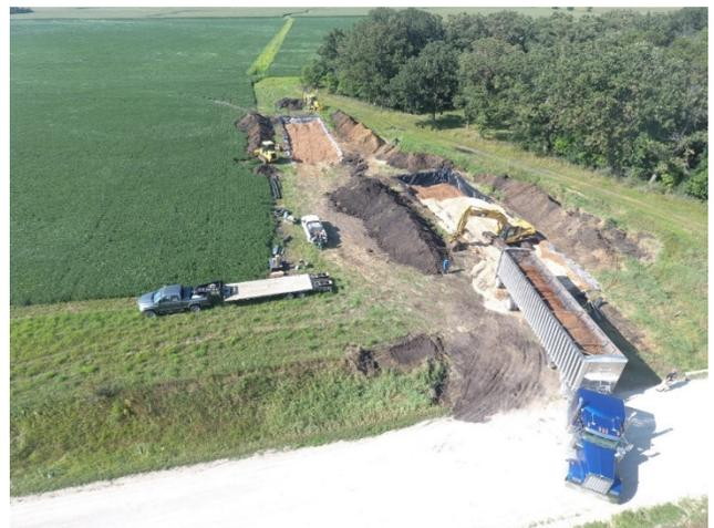
*A double bioreactor being installed on Mark and Eric Jellum's farm. The area will be seeded with a diverse prairie mix in the spring, providing habitat for wildlife and beneficial insects.*
