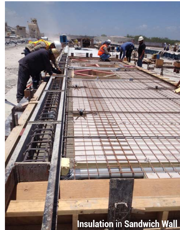
Steel Reinforcement in the Wall
