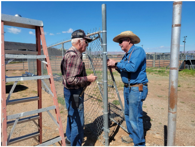
Gary & Steve installing a gate at the V.V. Fairgrounds.
