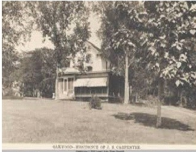
Figure 1 West face circa 1913 from book "Artwork of Des Moines" showing awnings and screened in porch.
