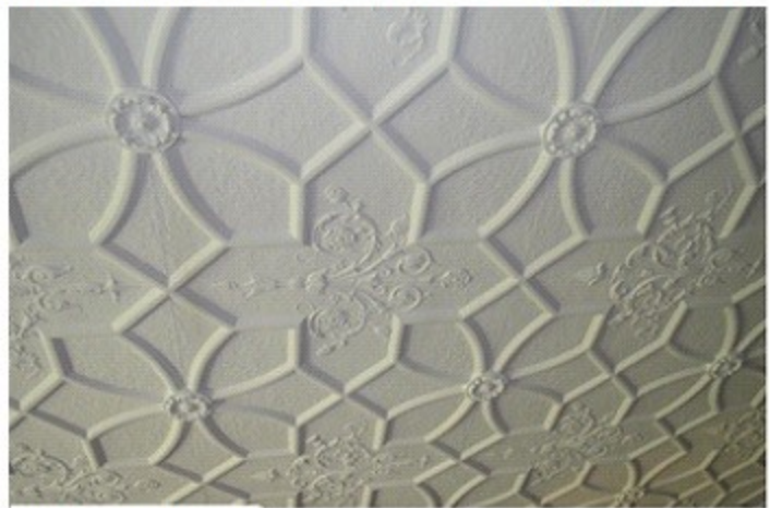
Figure 2 Great room ceiling.
