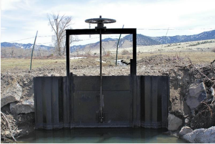
Headgate looking downstream
