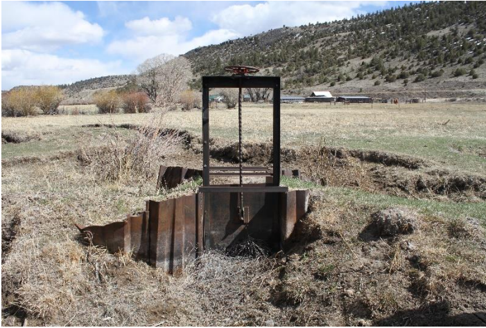
Headgate looking downstream
