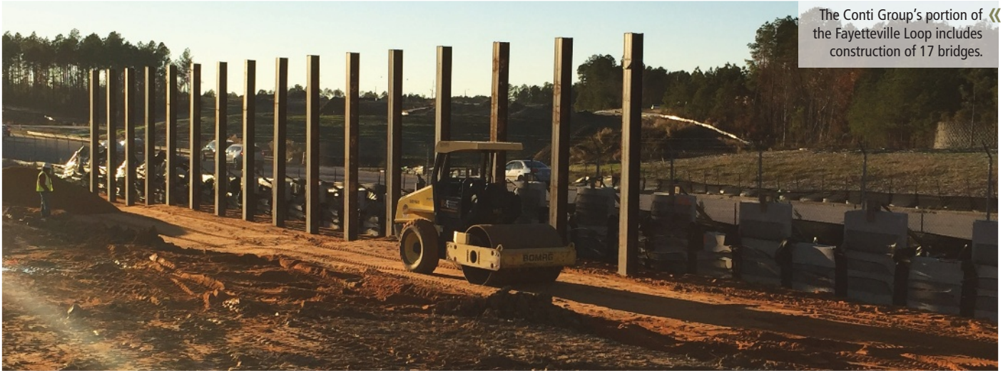
A mile-long sound barrier and visual barriers are being installed along portions of the highway.
