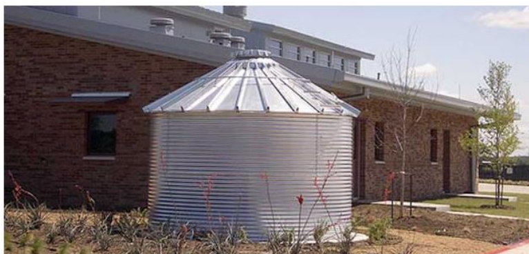
Photo: "IWS - watercache.com"; 5600 gallon commercial rainwater collection system for LEED Gold rated fire station in Denton, Texas. Rainwater is used to irrigate native plant landscaping around the station.
