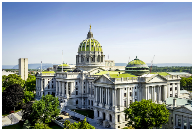
CAPITOL BUILDING IN HARRISBURG
