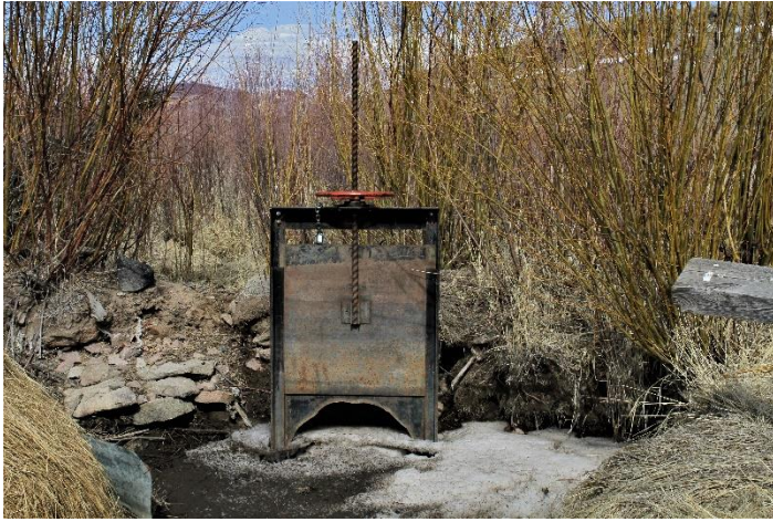
Headgate looking downstream
