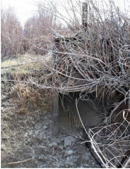
Headgate looking downstream
