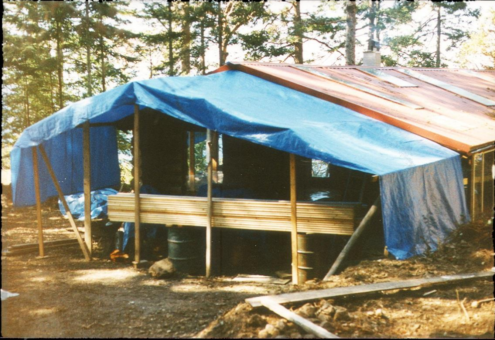
Temporary Storage For Flooring
