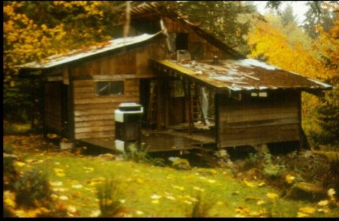
Kavadas Original Homestead By The Road Free For The Taking (To The Author) Everything Was Salvaged : Aluminum Roofing, Cedar Bevel Siding 1 x 10 Cedar Shiplap (Flooring And Other Interiors) Fir: 2 x 8, 2 x 6, 2 x 4 and 1/4 Ply.
