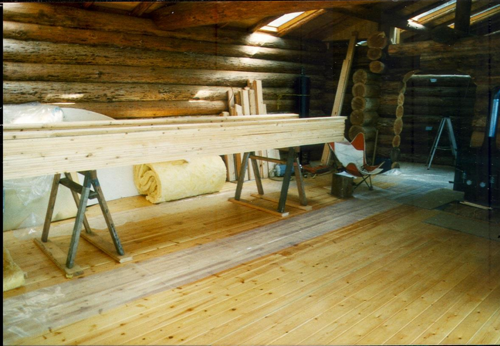
Working Out Of Finished West Section (Facing East)
