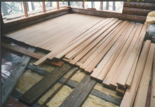
West Section Laying Out Flooring This Area Would Have Sixteen Foot Pieces Of Flooring Laid Without Lap Joints. The Butt Joints Would Be Under The Kitchen Counter. The Rest Of The Floor Would Be Lapped
