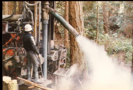
At Fifty Feet. Total Well Depth 105 Feet Yield Over Time: Approx. 1/2 Gpm
