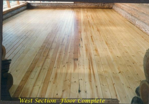
West Section Floor Complete With Three Coats Of Plastane (Polyurethane)
