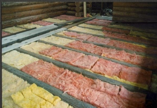
Insulating The West Section Floor. A 1/4" Galvanized Mesh Was Fastened To The Bottom Of The Floor Joists. The Joists On Average Were 6" Thick. Insulation Was Packed Between Joists To Floor Level
