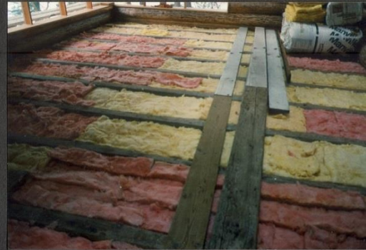
Insulating The West Section Floor. A 1/4" Galvanized Mesh Was Fastened To The Bottom Of The Floor Joists. The Joists On Average Were 6" Thick. Insulation Was Packed Between Joists To Floor Level
