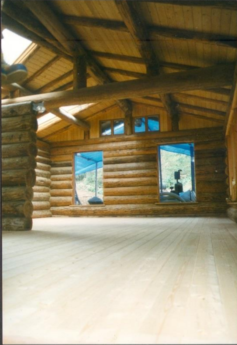
East Section Interior Finished Flooring East Section Facing East
