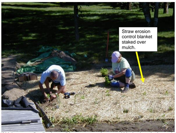
If high water or flooding is possible, a straw erosion control blanket is staked over the mulch prior to planting to prevent the mulch from being washed out. The blanket should have <u>bio-degradable</u> <u>netting</u>. Synthetic photo degradable netting often lasts many years and animals can get caught in the netting.
