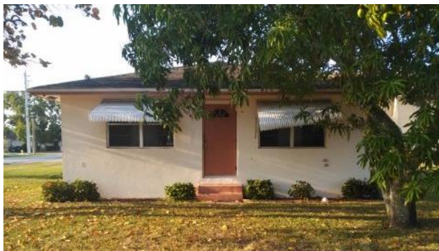
Current structure, Oakland Park, Florida.
