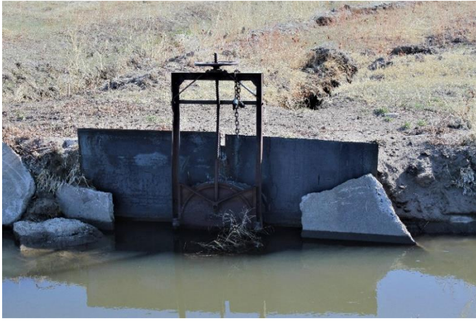
Headgate looking downstream
