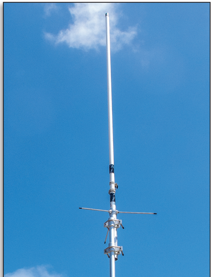
19. Completed antenna setup with antenna elevated.
