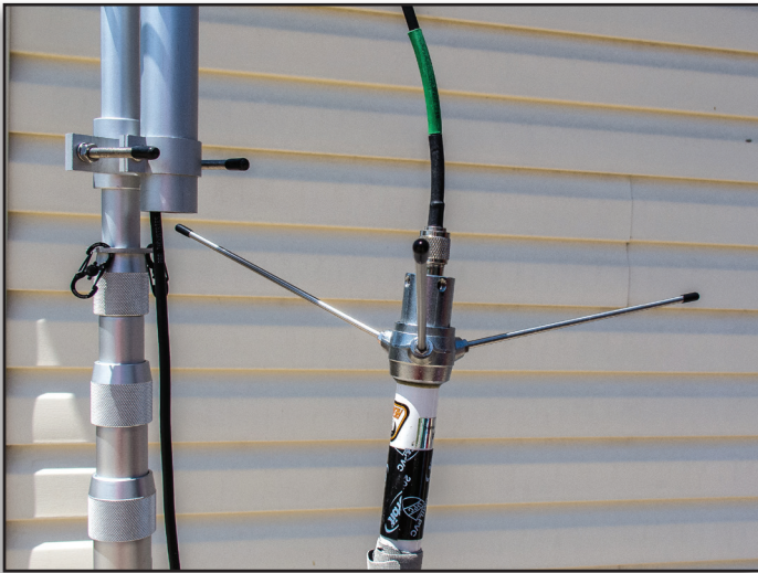
16. Antenna connected to coax before installation to antenna support bracket.
