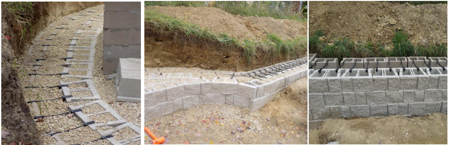
1st Course Lay Block & CMU's and Fill with Stone
