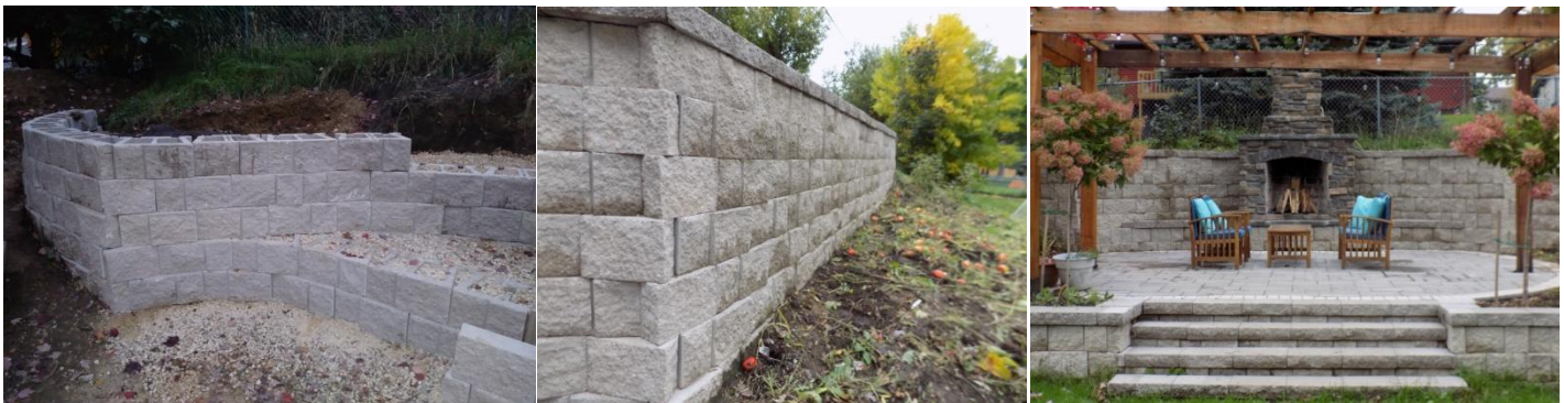
5th thru 7th Course Just lay block, backfill, compact
