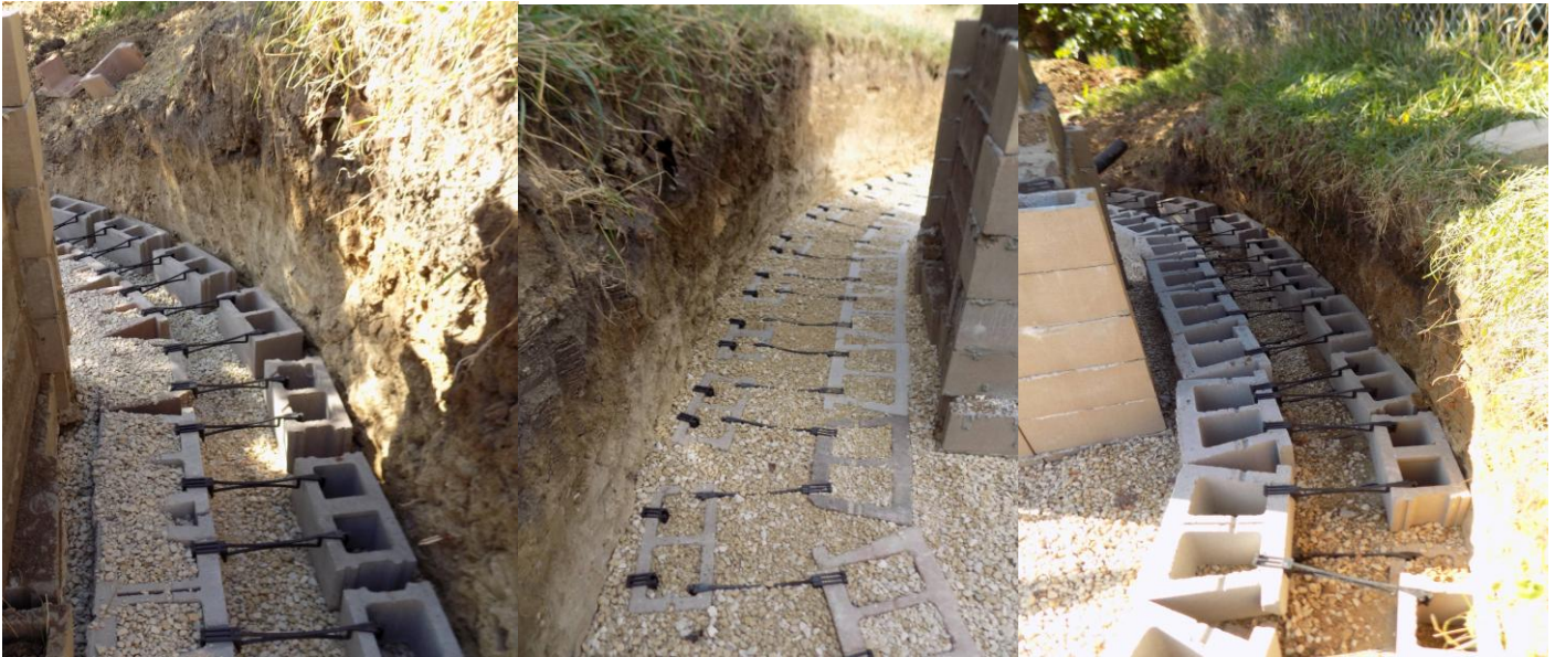
1st Course Lay Block & CMU's and Fill with Stone
