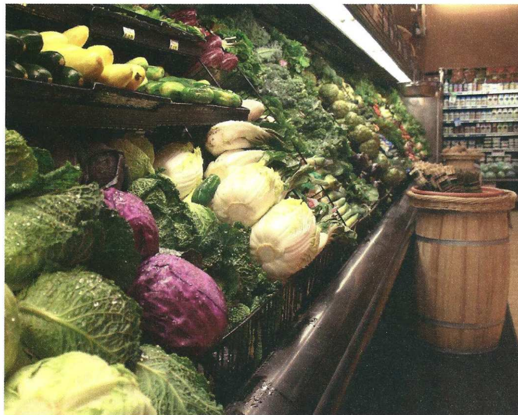
An open display case used to store fresh vegetables. The case has a drain, so the vegetables can be moistened by hand or with an automatic sprinkler. Courtesy KES Science and Technology Inc.
