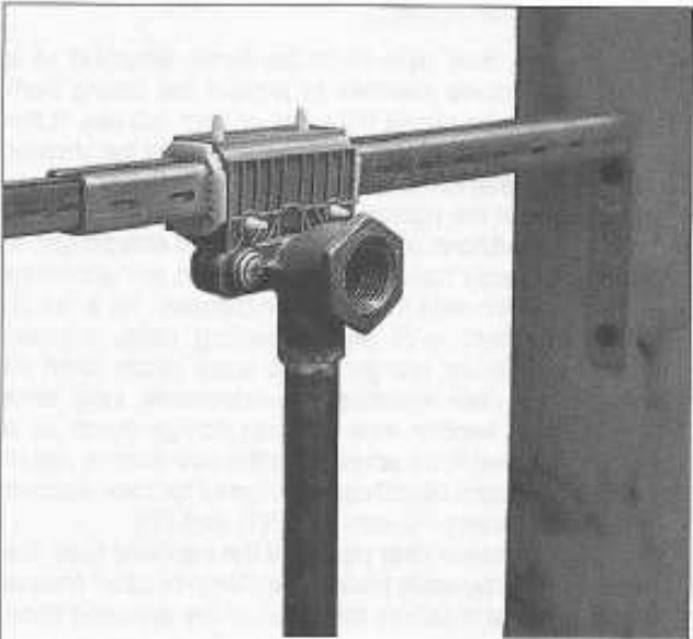
Figure 417.2(2) SPECIAL BRACKET FOR SHOWER RISER (Photo courtesy of Holdrite-Hubbard Enterprises)
