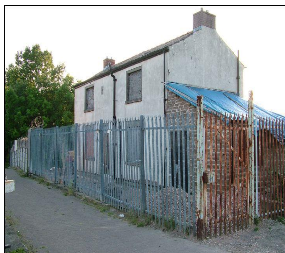
The Rose Bridge Lock Cottages being renovated
