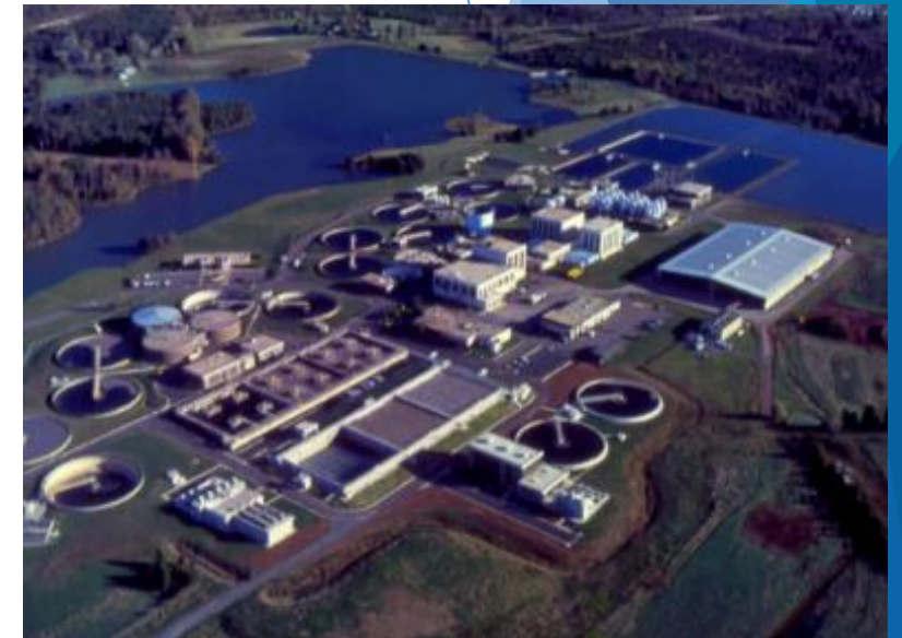
Millard H. Robbins Jr. Water Reclamation Plant Centreville, VA (UOSA)
