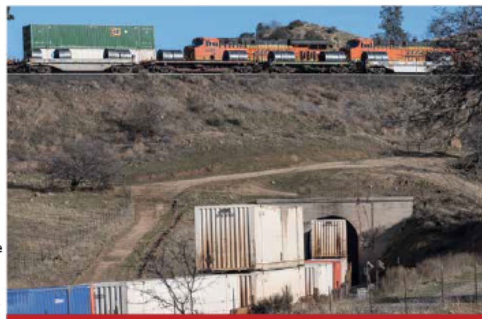
Train Exiting Tunnel
