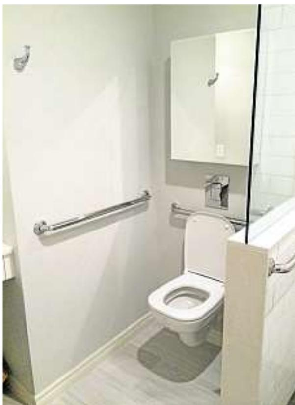
A wall-mounted toilet allows for the foot rests of the wheelchair (and the user's feet) to easily glide underneath and for more circulation space in the bathroom.
