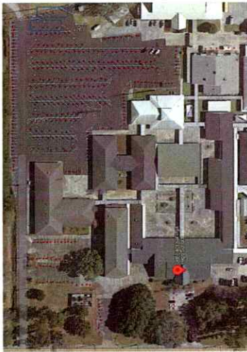
Area "C" - North side of High School and West of Main Building 7 van accessible parking spaces after lot is re-strip
