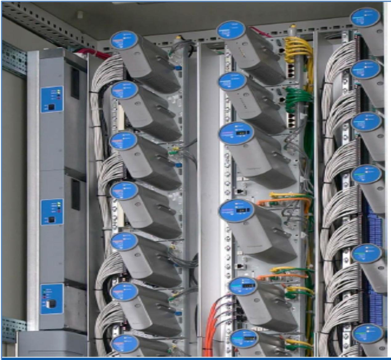
Honeywell Soft Configurable Universal Process I/Os in a Universal cabinet design
