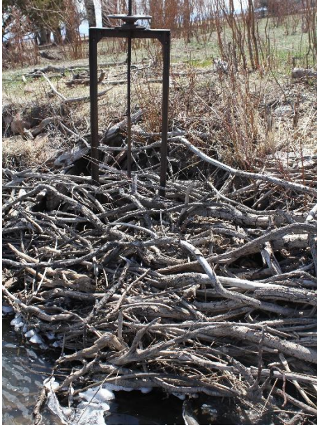
Headgate looking downstream
