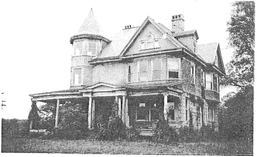
Daniel Carroll's mansion still stands at Alberene, though the years have taken a heavy toll. The house is now being restored by a Charlottesville businessman. (Author)
