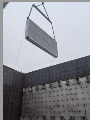
Baffles Replaced Through Open Stack
