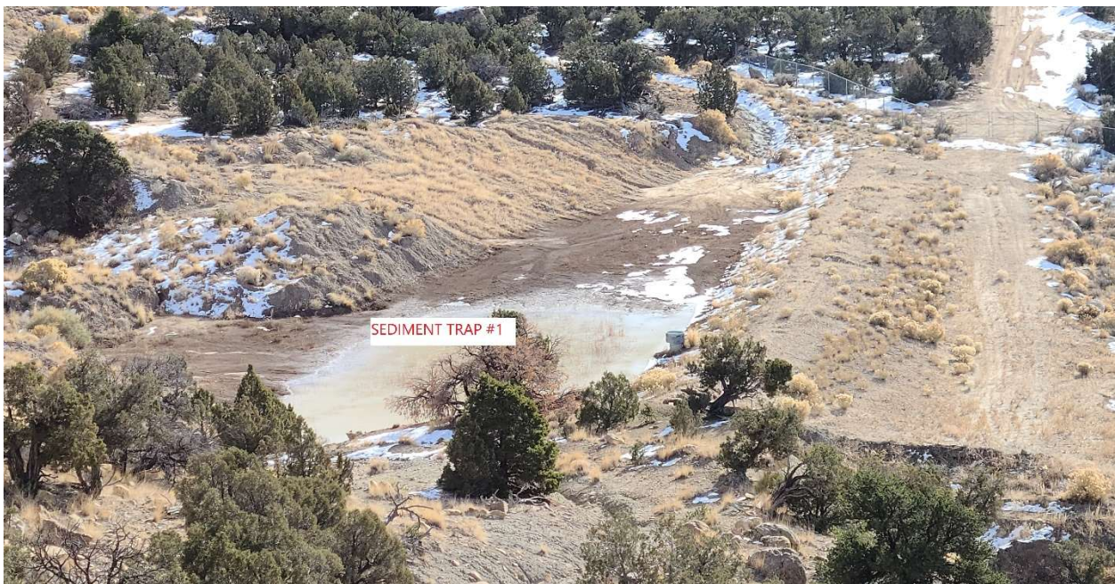
Sediment Trap #1 is has some water/ice water flows from trap #1 to pond 018 in normal open condition
