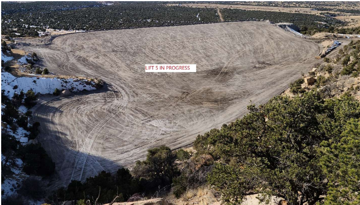
SCA#2 Ash Landfill – looking westerly Lift #5 in progress
