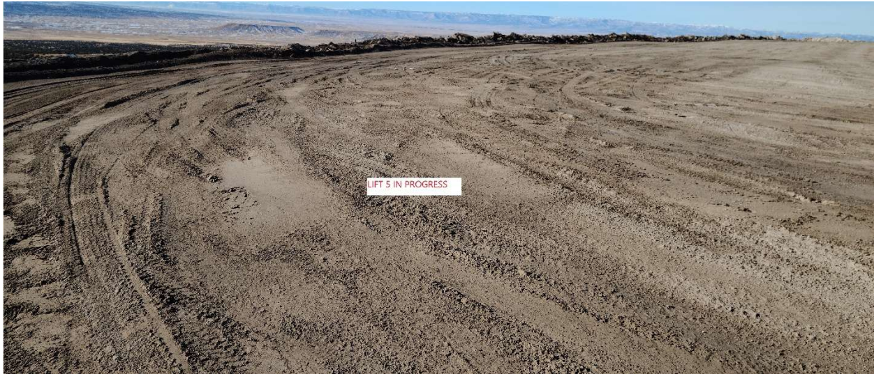
Lift #5 – in process – photo looking northwest
