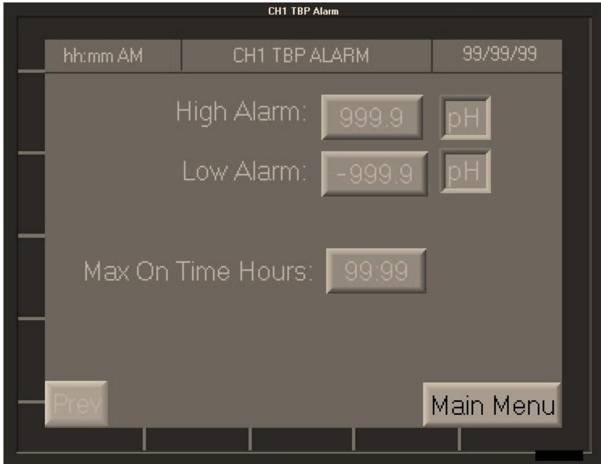
Figure 13: TBP Alarm Setup Screen
