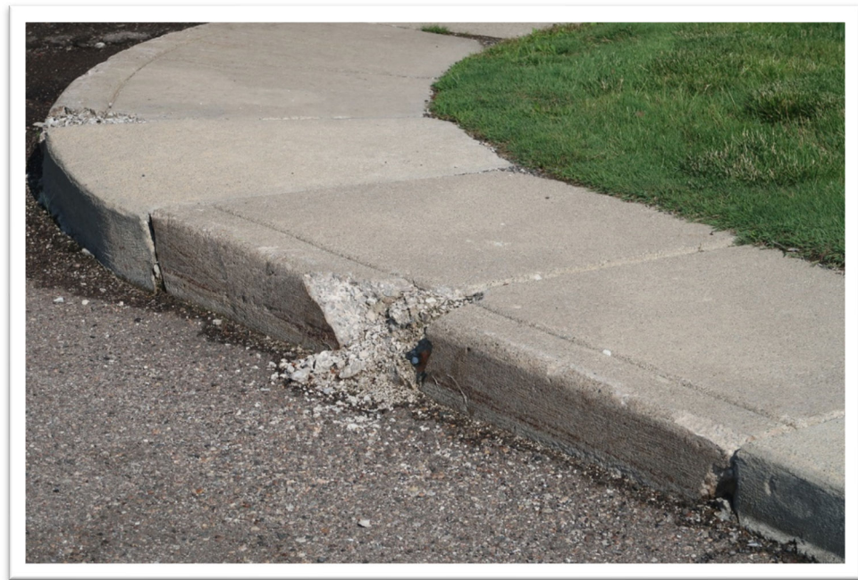
Photograph 28: Typical view of concrete sidewalk
