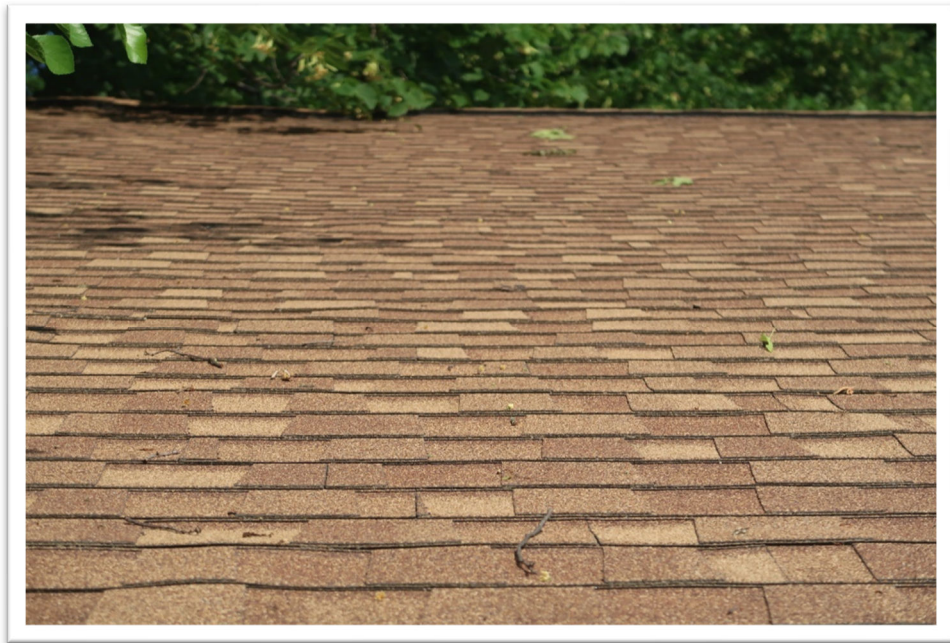
Photograph 49: Typical view of clubhouse asphalt roof shingles
