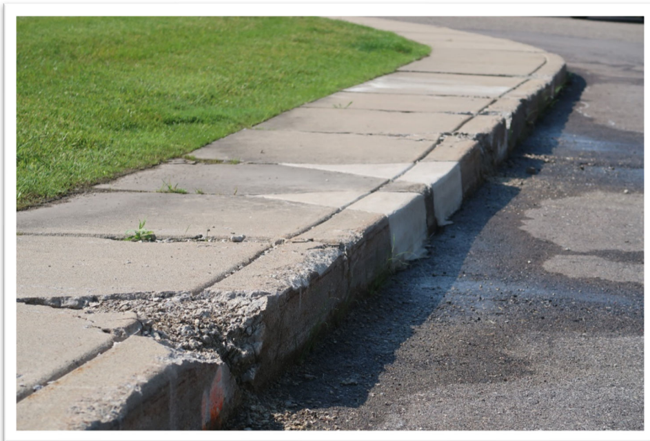
Photograph 30: Typical view of concrete sidewalk
