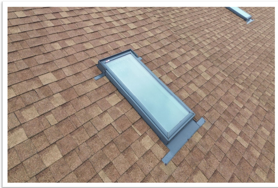
Photograph 15: Typical view of skylight
