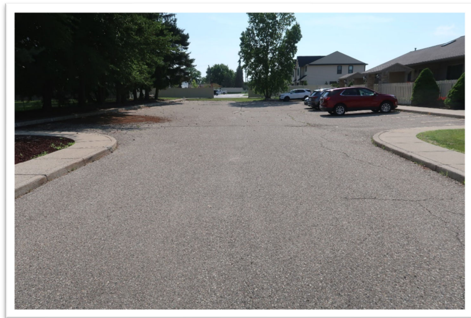
Photograph 34: Typical view of asphalt streets – Alexandria Court
