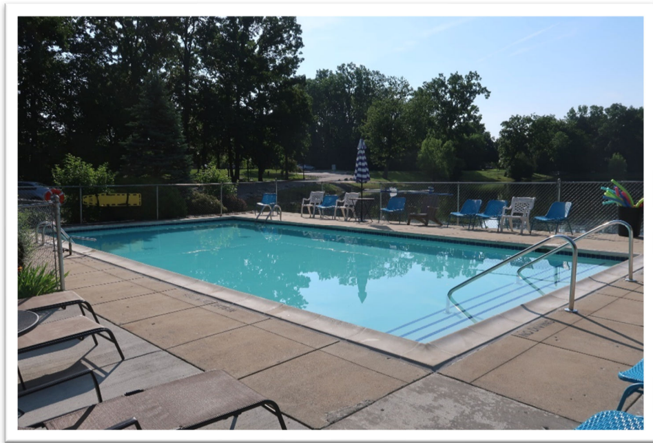
Photograph 55: Typical view of pool area
