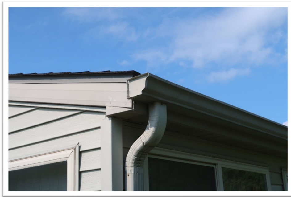
Photograph 13: Typical view of aluminum gutters & downspout – Newer model
