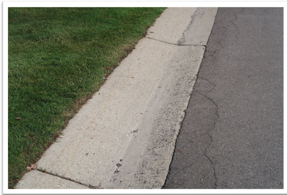
Photograph 31: Typical view of concrete curb
