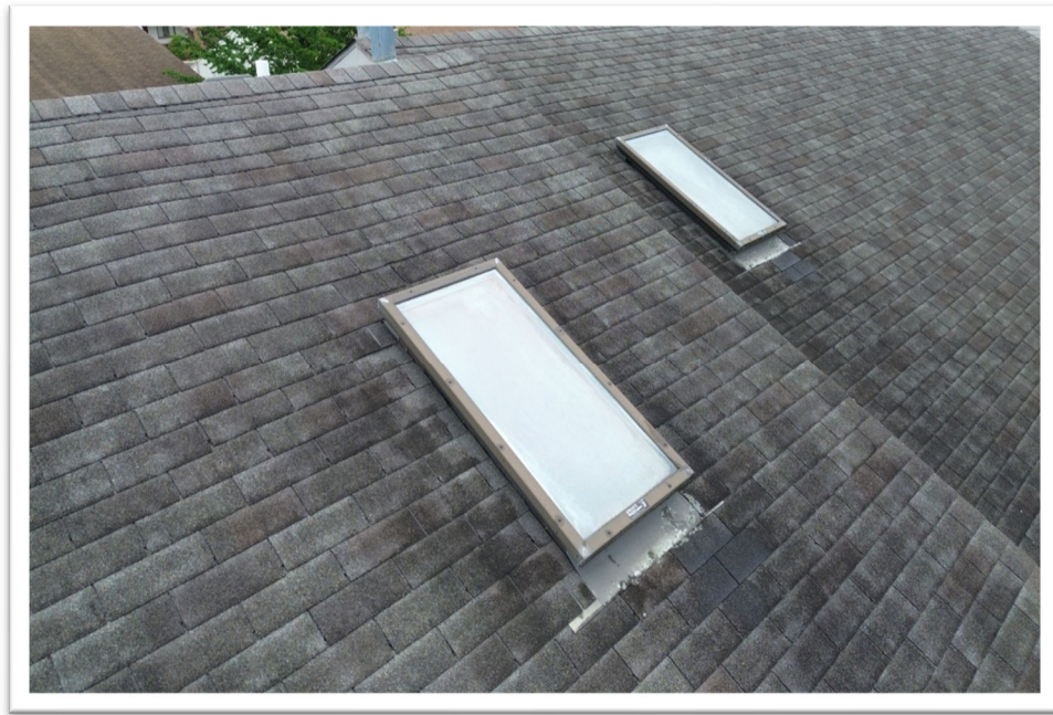
Photograph 17: Typical view of skylights
