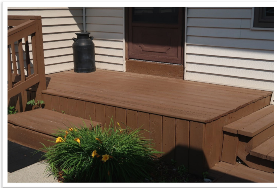
Photograph 25: Typical view of wood porch
