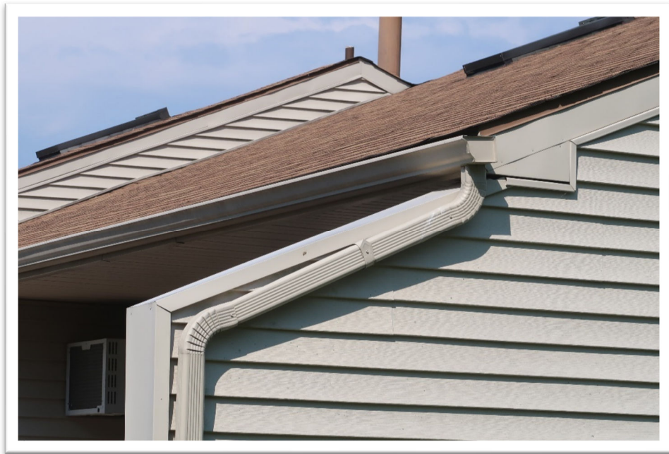
Photograph 11: Typical view of aluminum gutters & downspout – Older model
