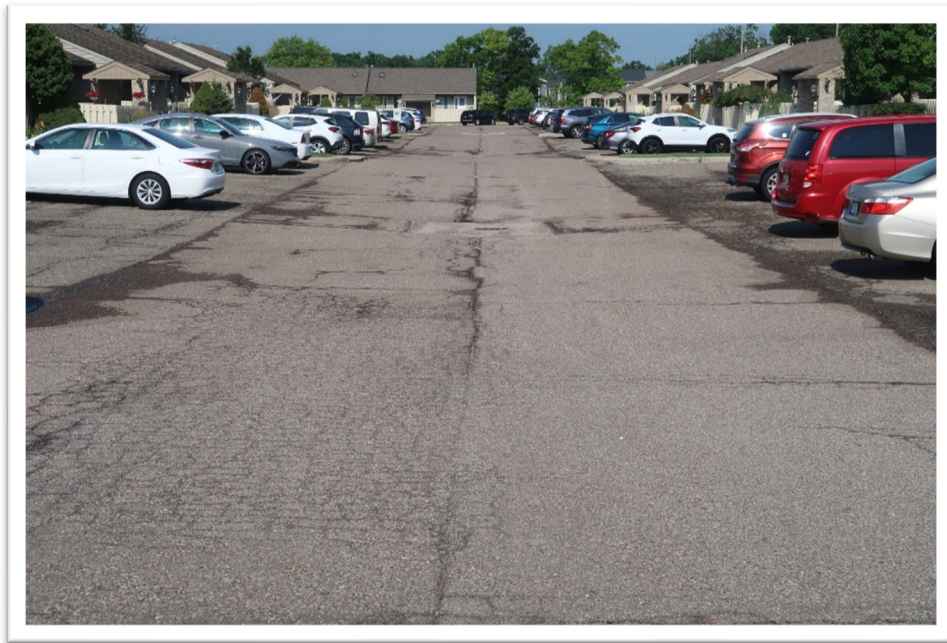
Photograph 33: Typical view of asphalt street – Arlington Circle
