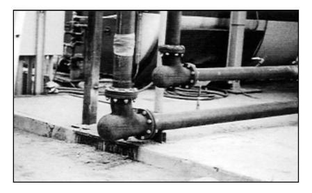
Smart Elbow<sup>™</sup> ends elbow wear problem in paving plant.
