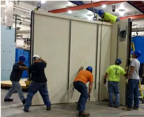
FIGURE 10: Placing a straight section of wall and connecting it to a corner section.
