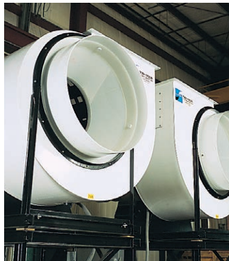
Dual fan set-up prior to installation of duct.
