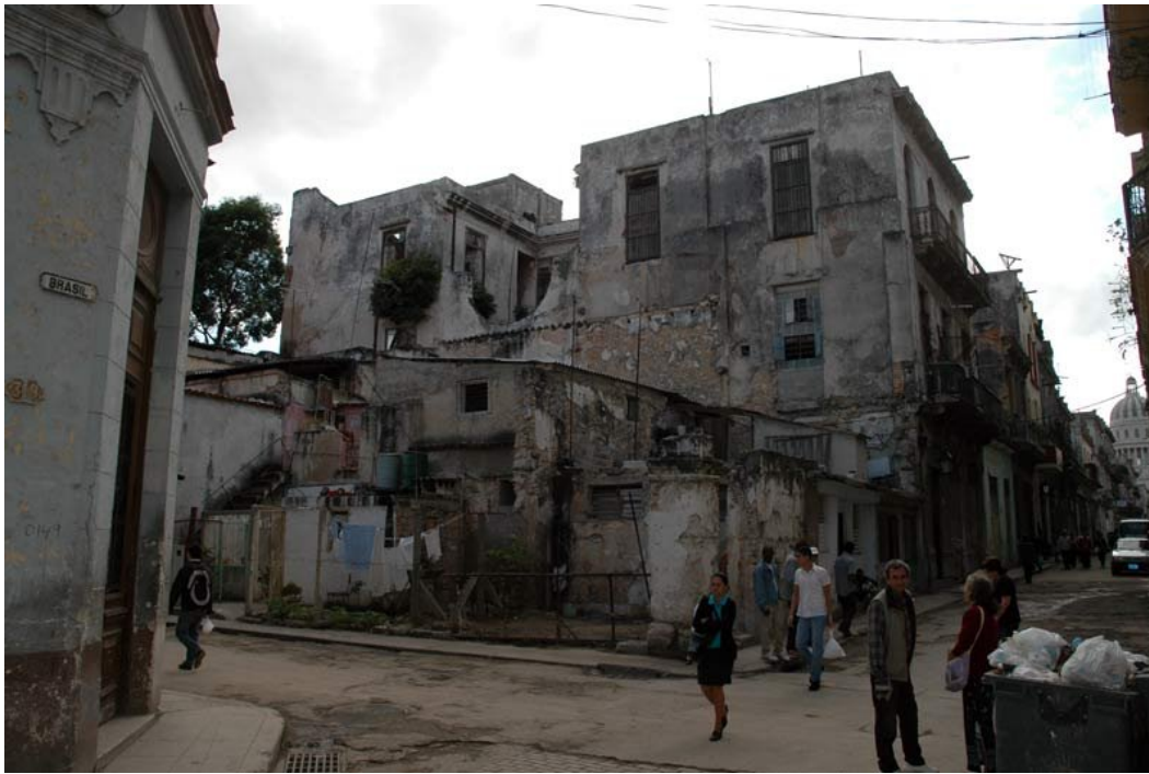
Image 6. Collapsing house in Old Havana. (Preservation Nation, 2011)
