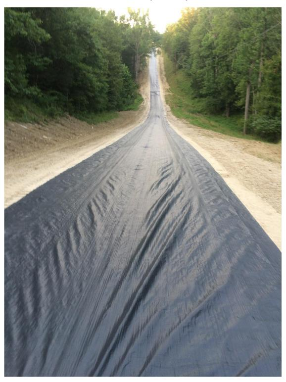
Attached is a picture of roller coaster hill after the road was dug up and ledge rock removed. The road was then rolled and the sides were then ditched to keep the water off the road. This
