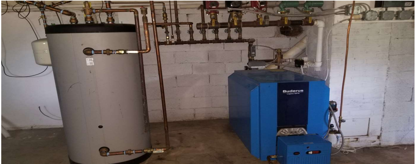
5 zoned heating and easy to get to automatic shut off valves
