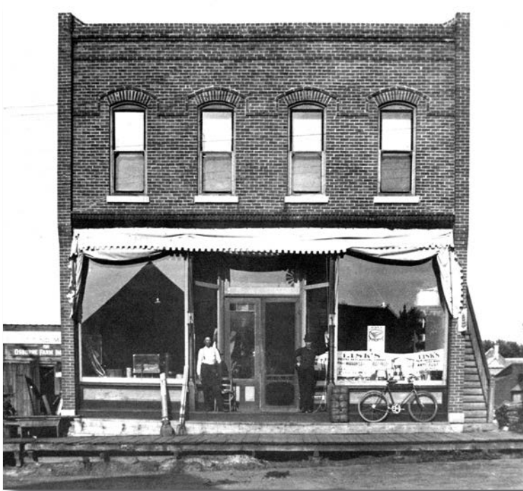
Note the large, oversized display windows, the bulkhead below and the retractable, canvas awning above.
