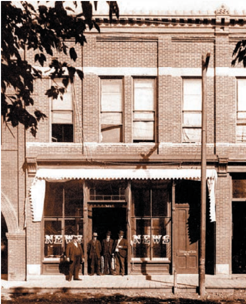
Turn-of-the-century photograph of the Northfield News Building, 311 Division Street. Large expanses of plate glass were commonly used to provide day-lighting and accommodate ample display. Note the verticality of the original storefront fenestration.
