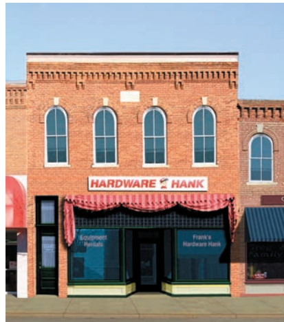
Flat signboards, low-profile projecting signs, painted lettering on the display windows and awning valance are appropriate.
