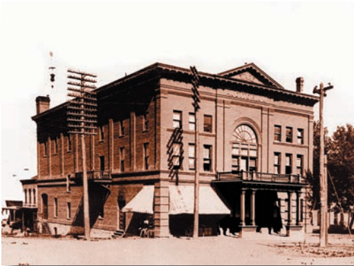
The Ware Auditorium displays a large, classical fan window, pilasters, fenestration symmetry, and originally had a formal balustraded portico entrance on the Washington Street facade.
