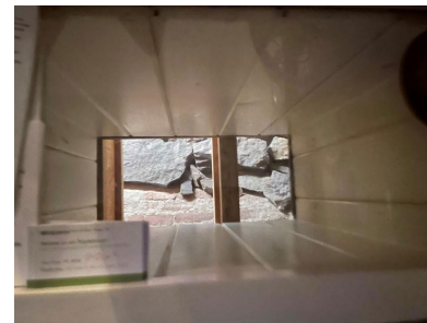
A view into the tunnel has been built from the first floor above.
