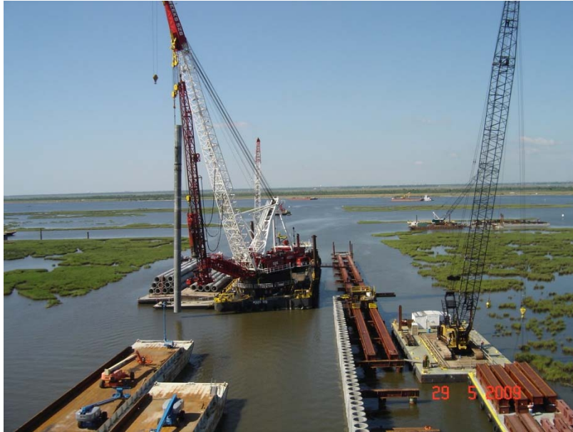
66" Cylinder Pile 144-ft Long
