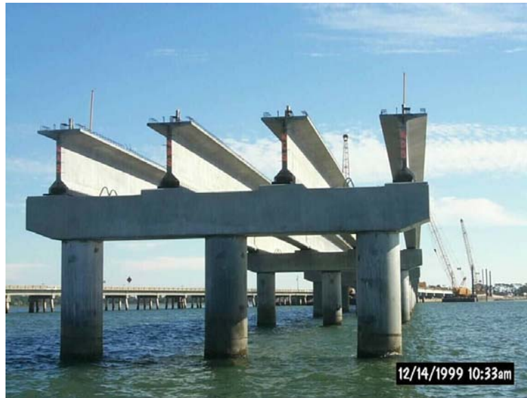
Bridge Bent with precast Cap
