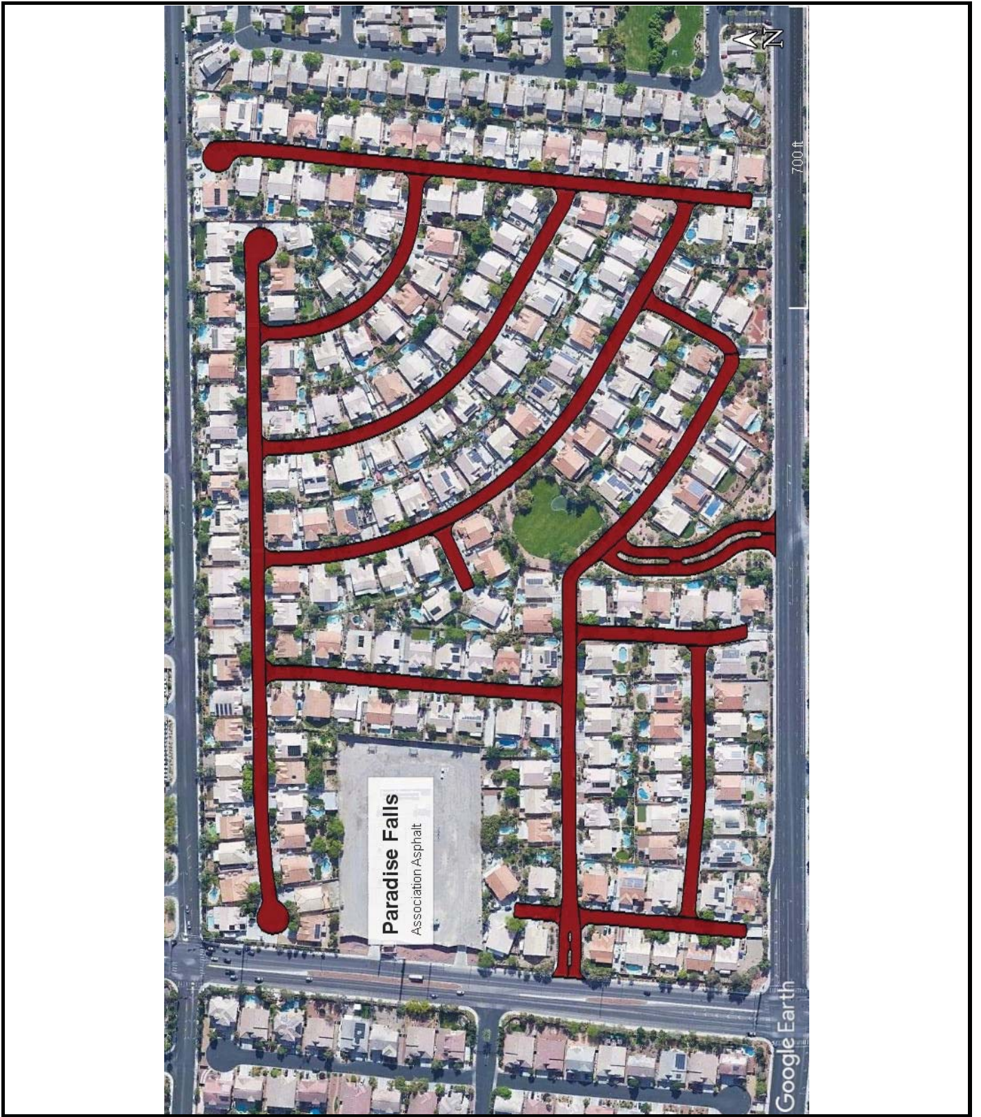
Association maintained asphalt.
