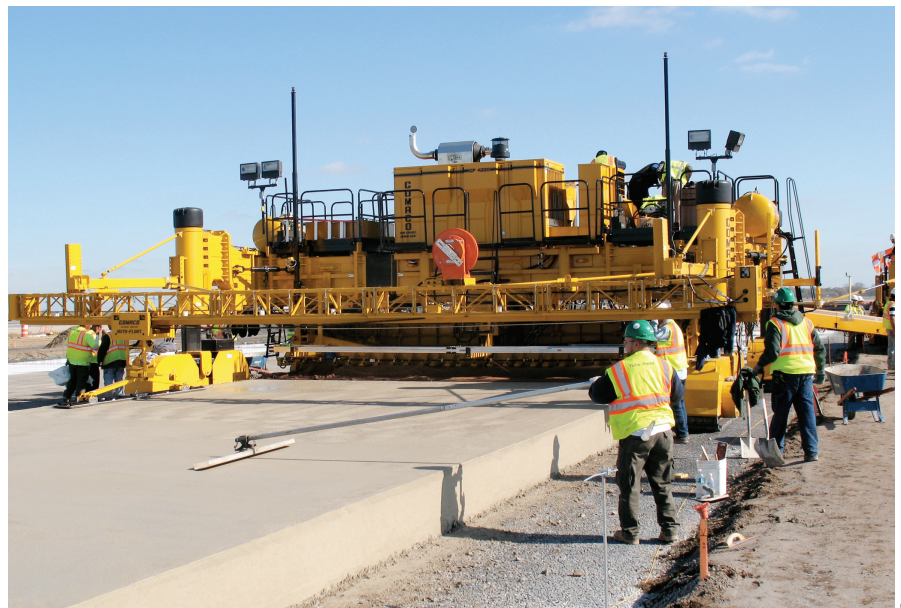
Note the two Leica prisms atop this four-track Gomaco paver.
