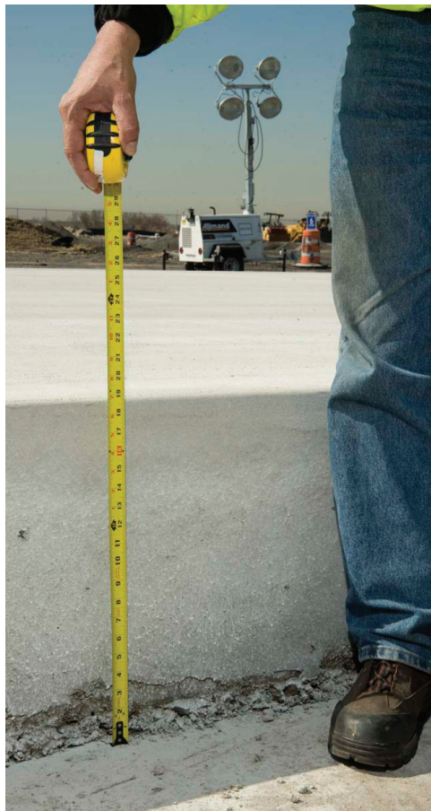
The concrete slab on the Bay Runway is 18 inches thick.
