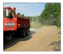
Scott Wipper eyeballs his truck's box to make sure he has unloaded the right amount of erosion stone at the Rush Lake Dam
