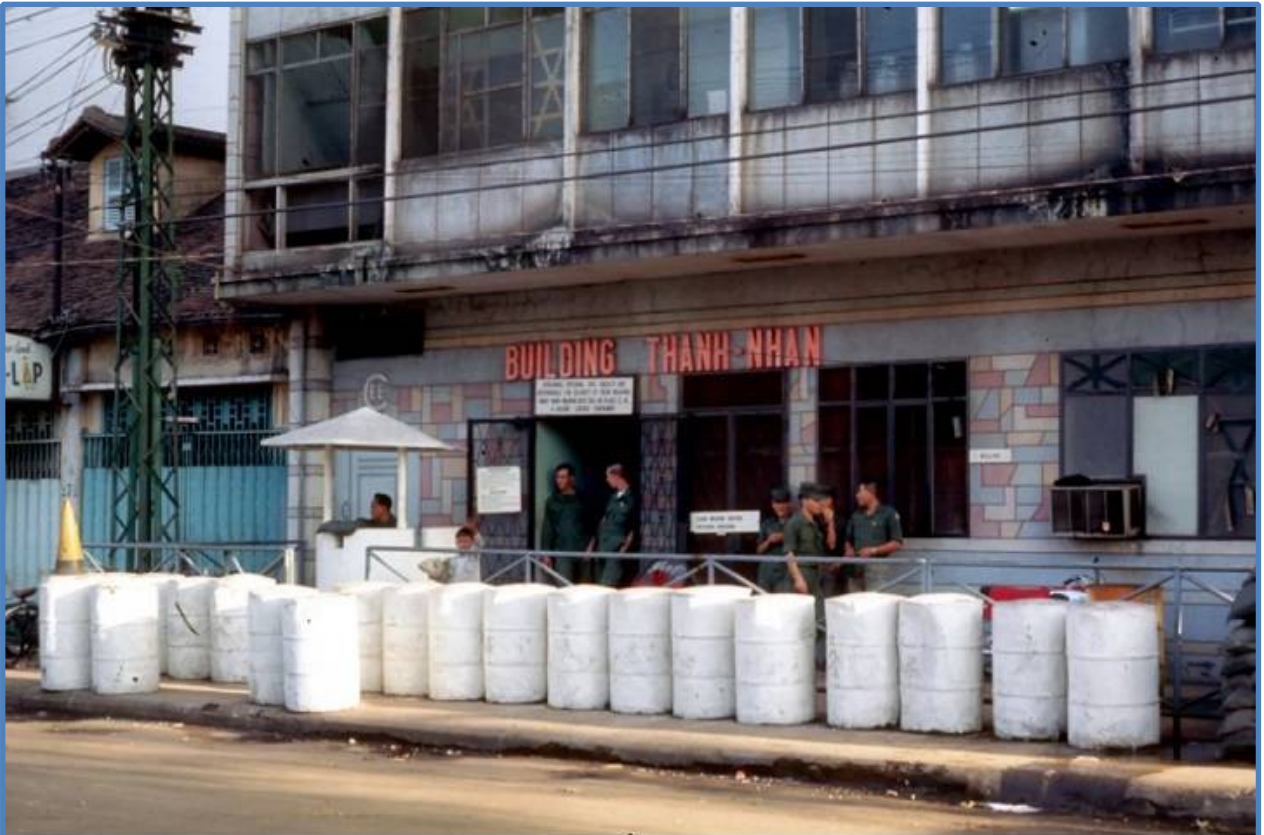
Barriers in front of the Walling BEQ
