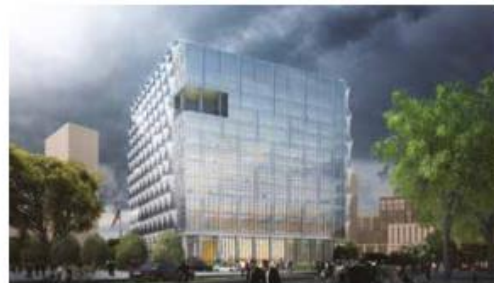
US embassy in Nine Elms, Battersea. The 11 storey cube-shaped building, one of the highest performing energy use and sustainability in the world
