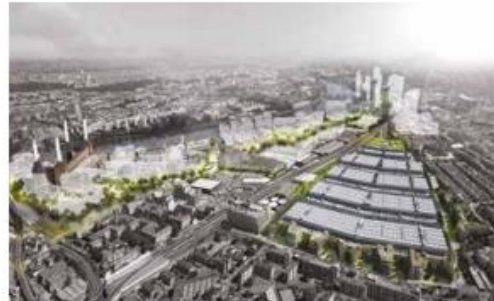
Nine Elms on the South Bank, will be one of London's greatest transformations, becoming an ultra-modern complex offering 16,000 homes and 25,000 jobs, schools, parks, culture and the arts, set over 196 hectares including the iconic Battersea Power Station
