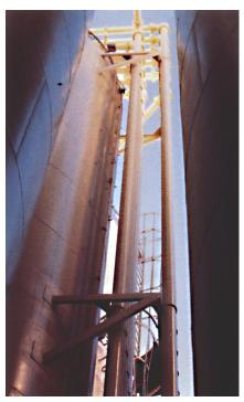
These 95' pipes were assembled on the ground and then stepped into their racks, greatly reducing costly crane time.
