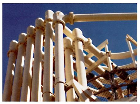
The compact design of the Smart Elbows<sup>™</sup> saves space the twelve 6" elbows shown here occupy the same space as a large desktop. They may also be rotated on their flanges for greater design flexibility and installation ease.
